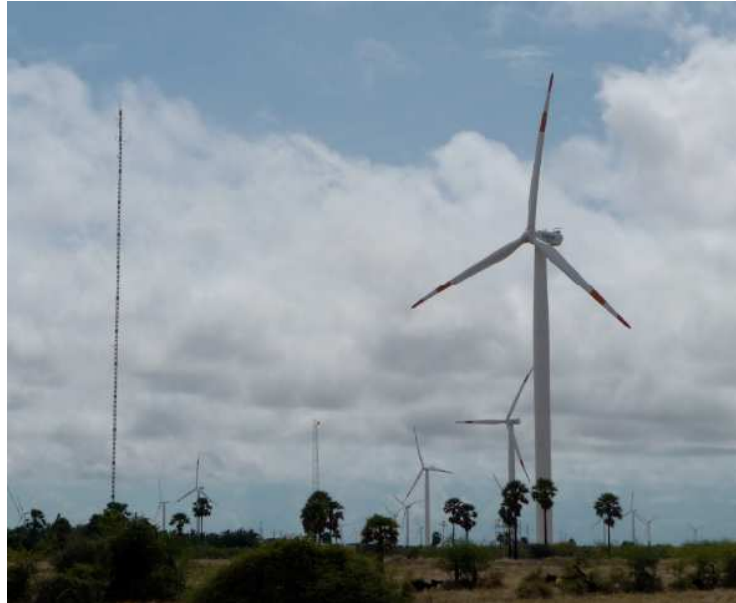
Figure 4-8: SUZLON S82 1500kW wind turbine situated nearby Sankaneri, Tamil Nadu in India
